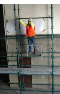
Figure 5: Photographic illustration of erection and dismantling using two erection platform options for a three plank wide scaffold. Note: scaffold is shown against a building, so guardrails only needed on external face. Toeboards and lower mid-rails omitted for clarity.
